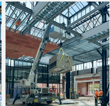
Photo of air handler installation at the mezzanine
