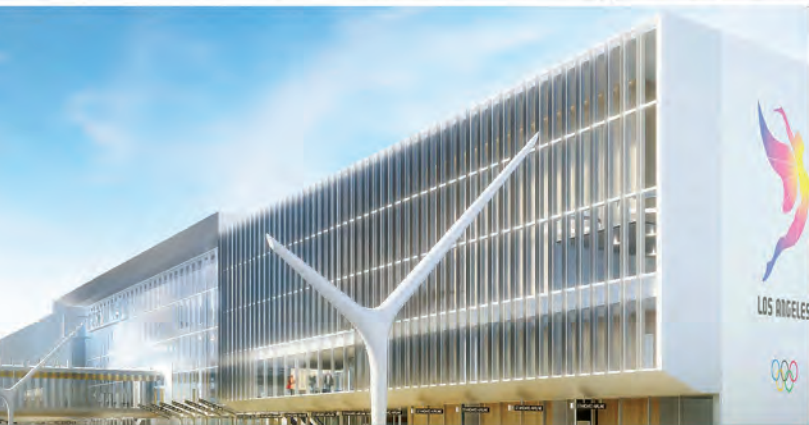
LAX Tom Bradley Int'l Terminal APM Interface (Design Build HVAC & Plumbing)
